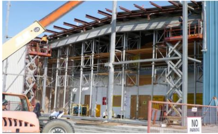
Main front entry steel framing is complete.
